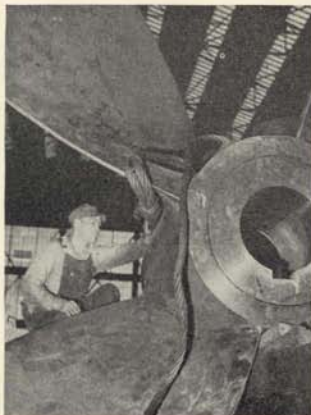
Ship propeller, cast in one piece, being lifted into place.
